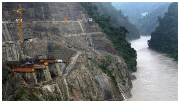
Lower Subansiri Hydroelectric Power Project site
